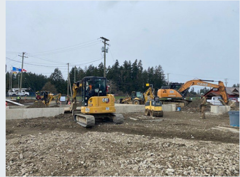
Foundation infill in progress – Feb 27 th .
