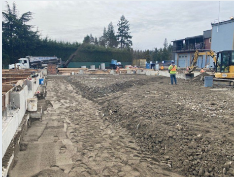
Foundation infill has begun – Feb 27 th .
