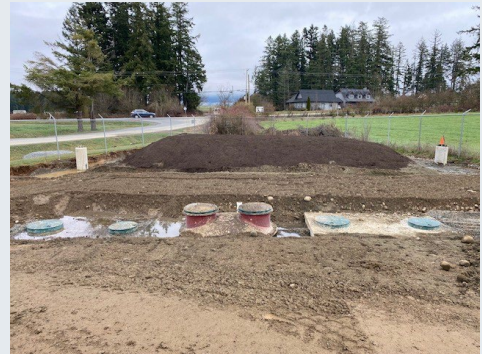
Septic system – Feb 23rd.
