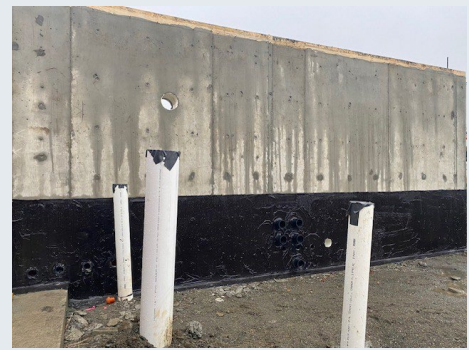
Damp-proofing is in progress.
