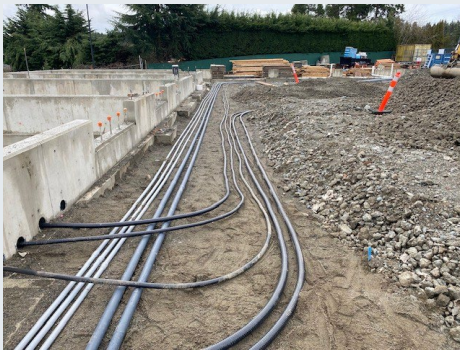
Below slab service piping install in progress.
