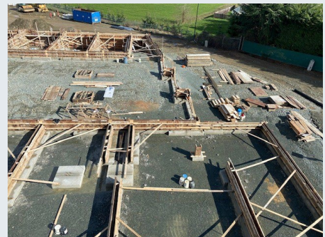
Foundation wall formwork – Feb 22nd.
