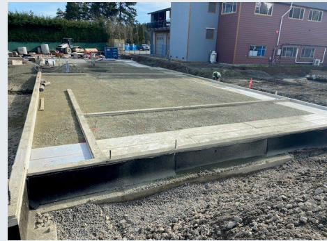
SOG prep in progress.
