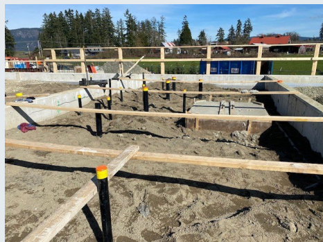
Plumbing rough-in in progress.
