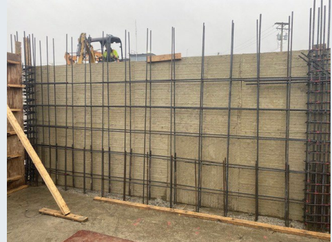
Stair tower South Elevation – level 1.
