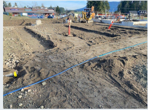
Trench drain recess prepping for installation.
