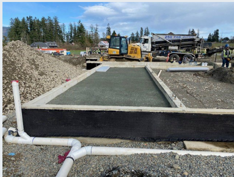
SOG prep in progress.
