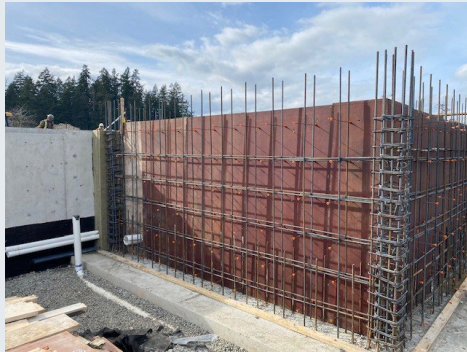
Stair tower formwork.
