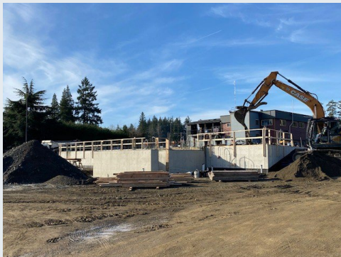
Concrete stair/hose tower.
