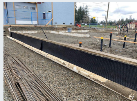
Damp=proofing and drainage mat.
