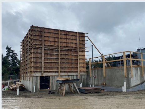
Stair tower formwork for 2 nd level.
