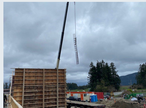
Rebar zone flying into stair tower
