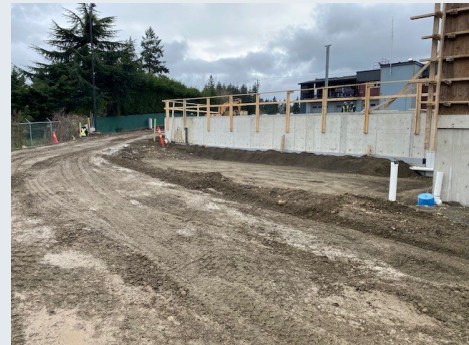
Tank location prepped.
