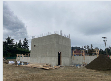
Stair tower exposed concrete.
