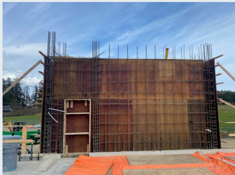
Stair tower level 2 reinforcing steel.
