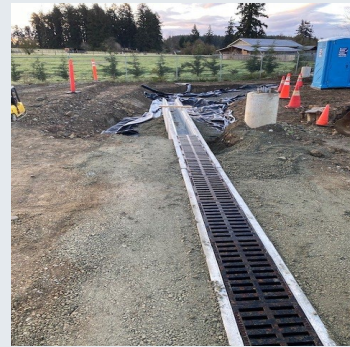
Trench drain and rain garden in progress.
