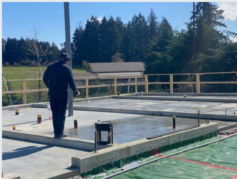
PentraSil 244 sealer install in progress.
