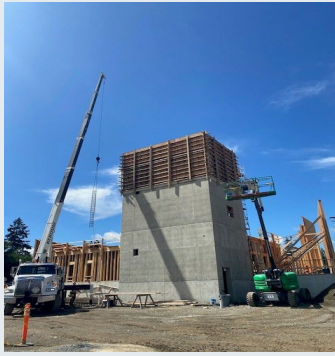
Stair tower – formwork and rebar in progress.
