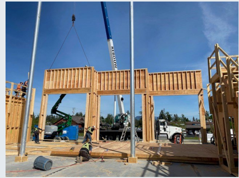
Exterior wall erection.
