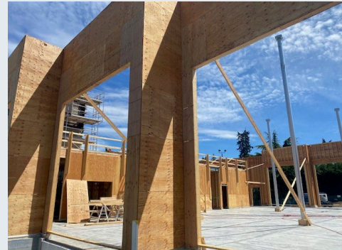
General – West elevation looking North.
