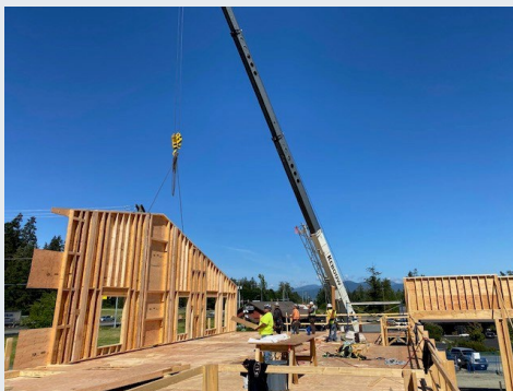
Crane lift of L2 walls.
