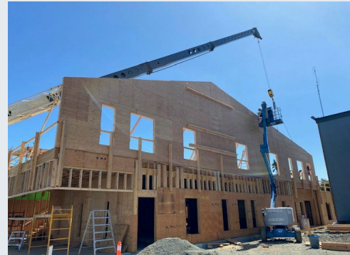
May 23rd - GL1.1 - L2 wall standing.
