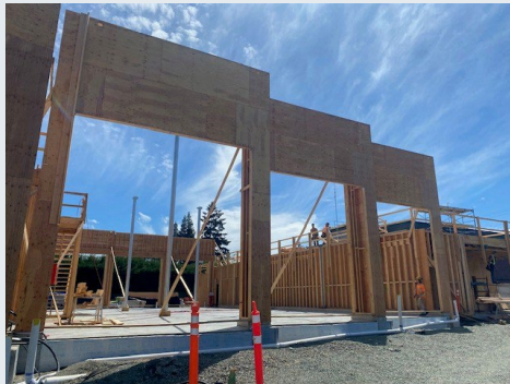
General – West elevation looking South.
