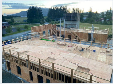
General – May 22nd – GL1.1 wall ready to stand.
