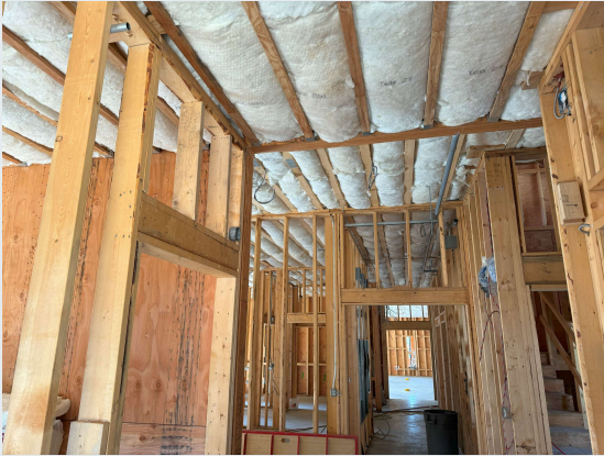
L1 South ceiling insulation complete / drywall commenced
