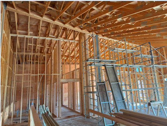
L2 South interior framing near complete
