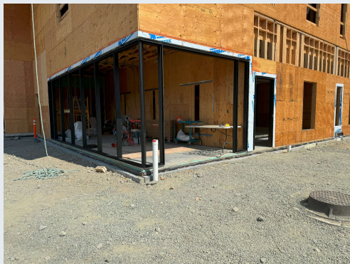
Aluminum frames and vinyl window mockup progressing
