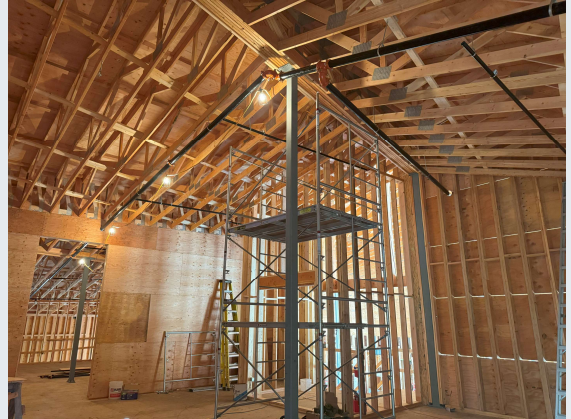
L2 North sprinkler installation commenced
