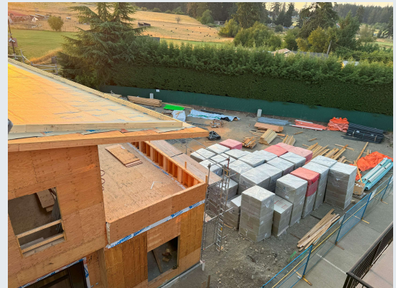
Roof insulation onsite.
