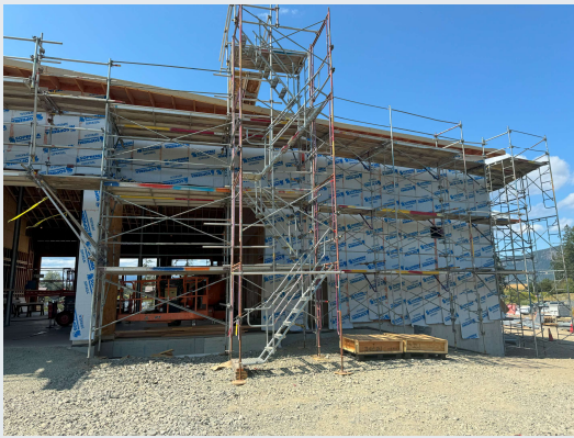
Wall membrane progressing East
