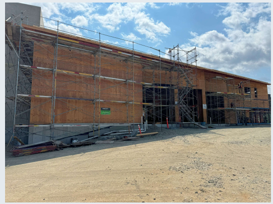
Envelope access scaffold on West progressing
