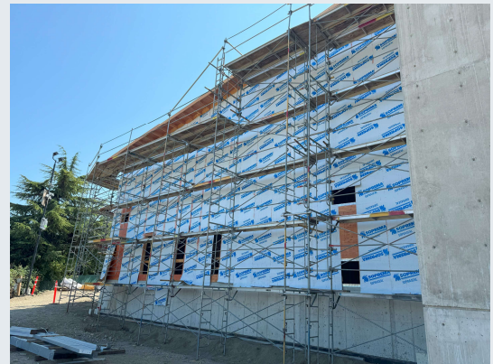
Wall membrane progressing North
