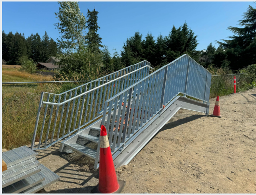
Hose tower stair pre-fab started
