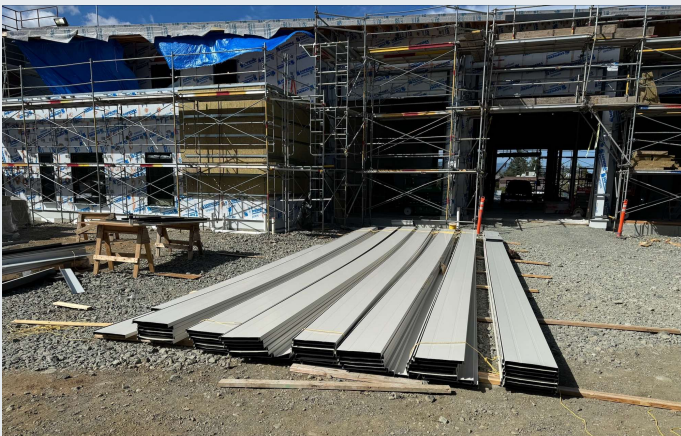
Roof metal prepared for install
