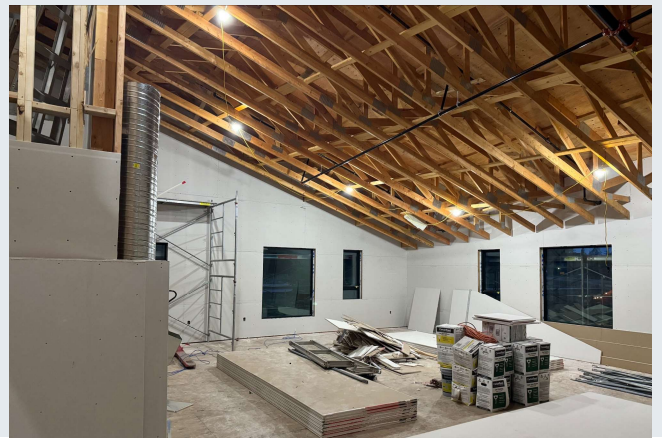
Fitness Area drywall progressing
