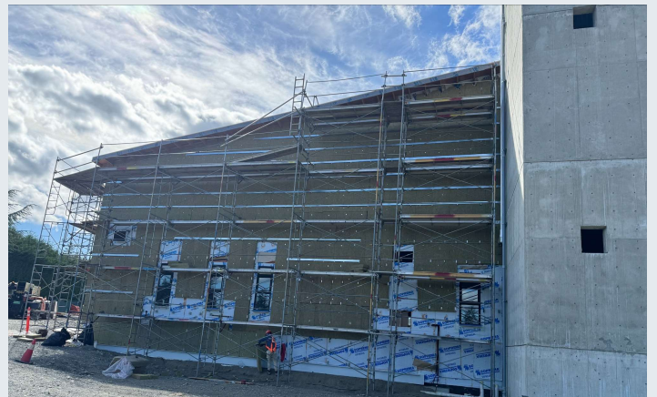
Exterior insulation & membrane progressing
