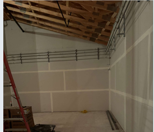
Drywall fire taping progressing
