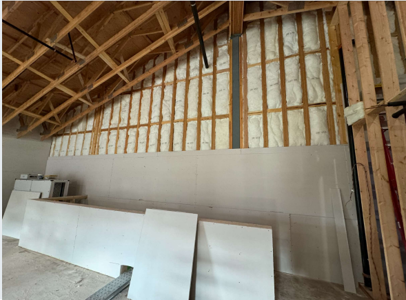
Fitness Area drywall progressing
