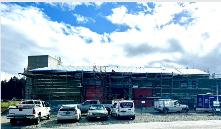
Roof metal install commenced
