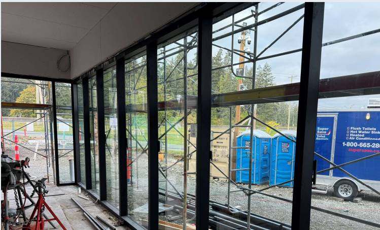
Curtain wall glazing installed
