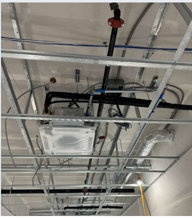
Ops side heating and cooling install progressing
