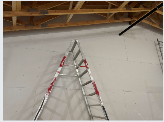
Fitness Area boarding completed
