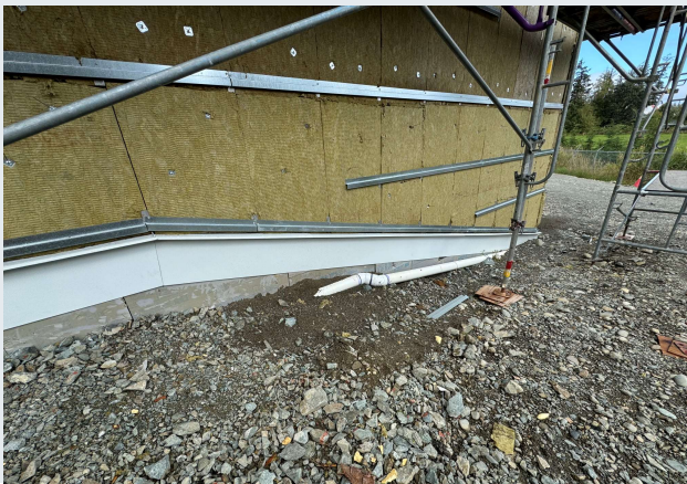
Base flashing install progressing
