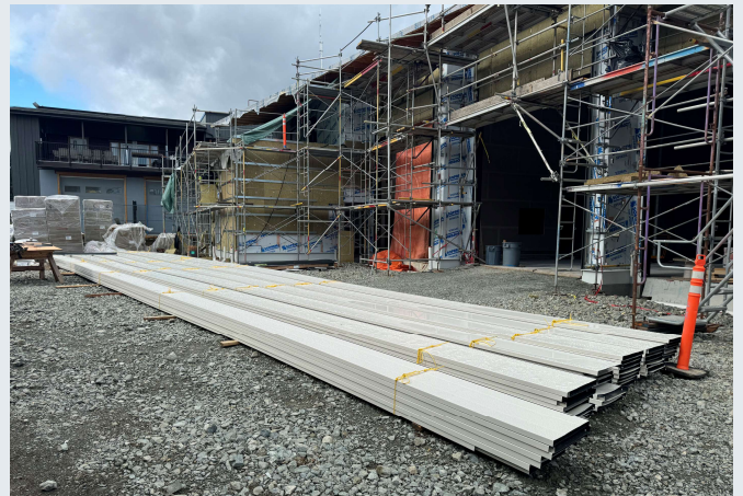
Roof metal prep progressing
