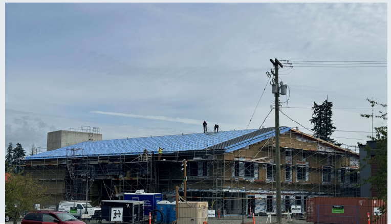
Exterior envelope progressing
