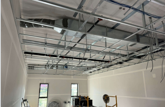
Ceiling drop framing progressing
