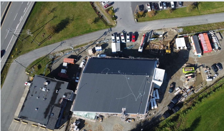
Slope roof substantially complete
