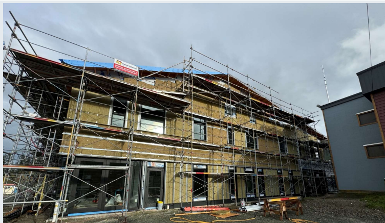
Exterior insulation nearing completion
