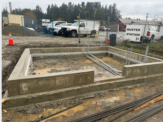
Pump Building foundation placed
