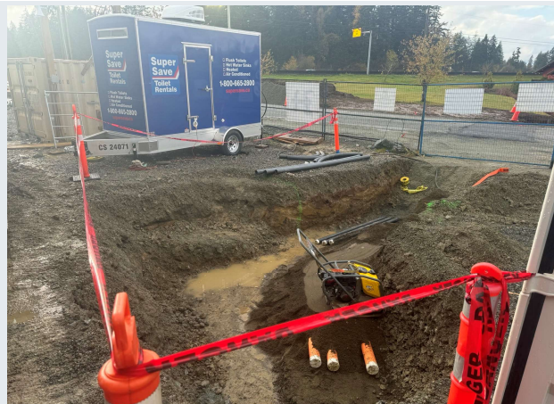
PMT underground works progressing
