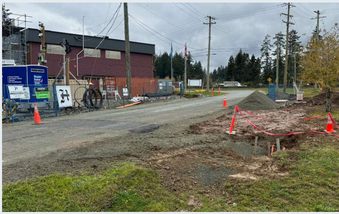
Offsite Hydro, Telus & Rogers installs near complete
