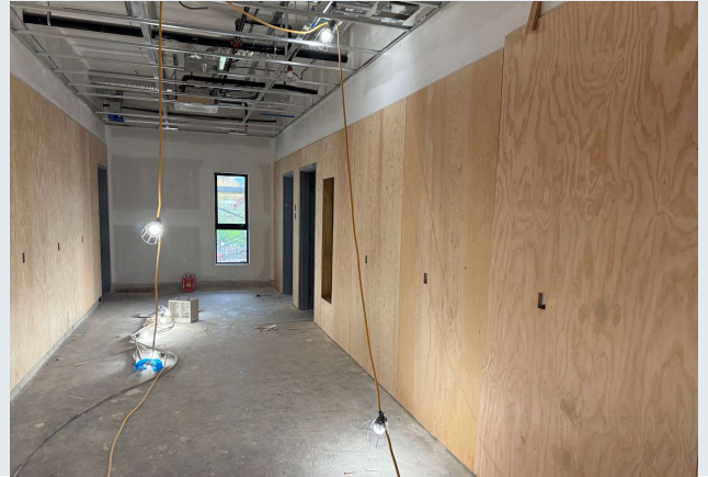
Interior works progressing
