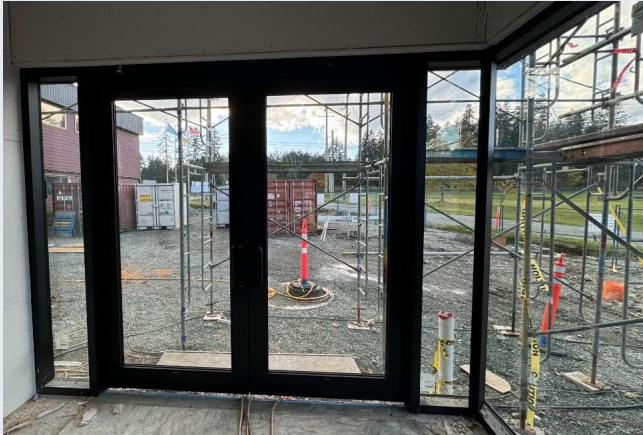
Curtain wall glazing near complete
